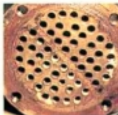
After Installation of ED 2000
